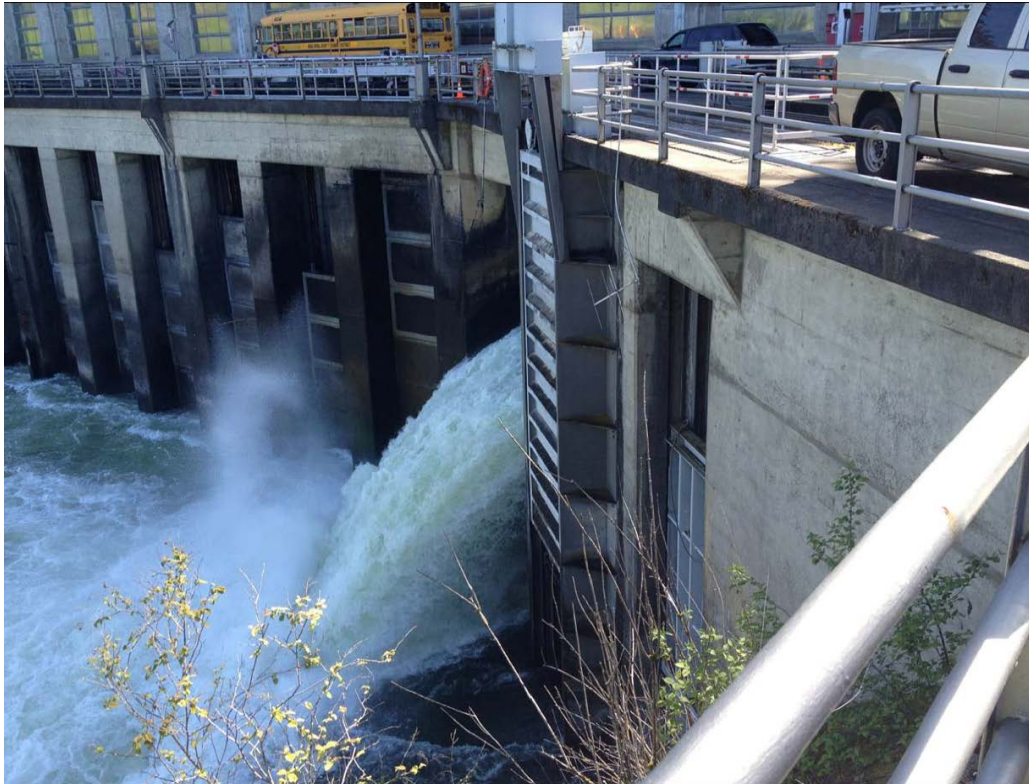
Figure 6-4. B1 ITS Outfall Pass-Through Antenna
