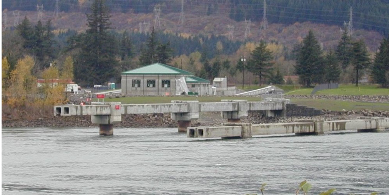
Figure 6-9. JBS Outfall Piers
